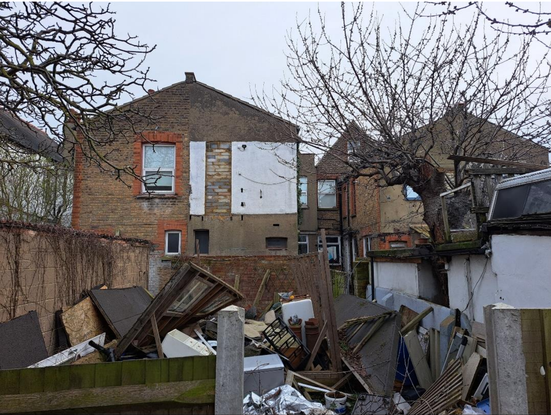
Rears of 77-83 West Road/ remnants of demolished outbuildings forming application site
